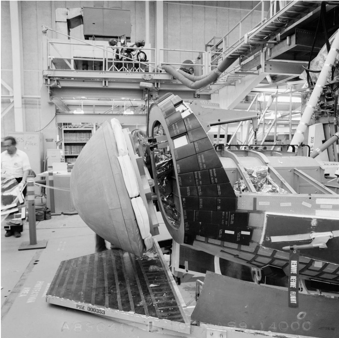
Figure B-43. Installation of Discovery's nose cone in High Bay 2, AFP 42, March 8, 1983. Source: NASA, Johnson Space Center Image Repository, JSC2010-03441.
