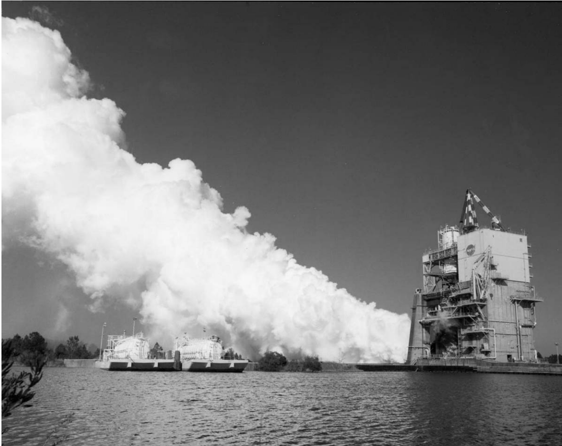
Figure C-16. A “Return to Flight,” Phase II SSME undergoing testing on Stand A-1, camera facing northeast, 1988.
