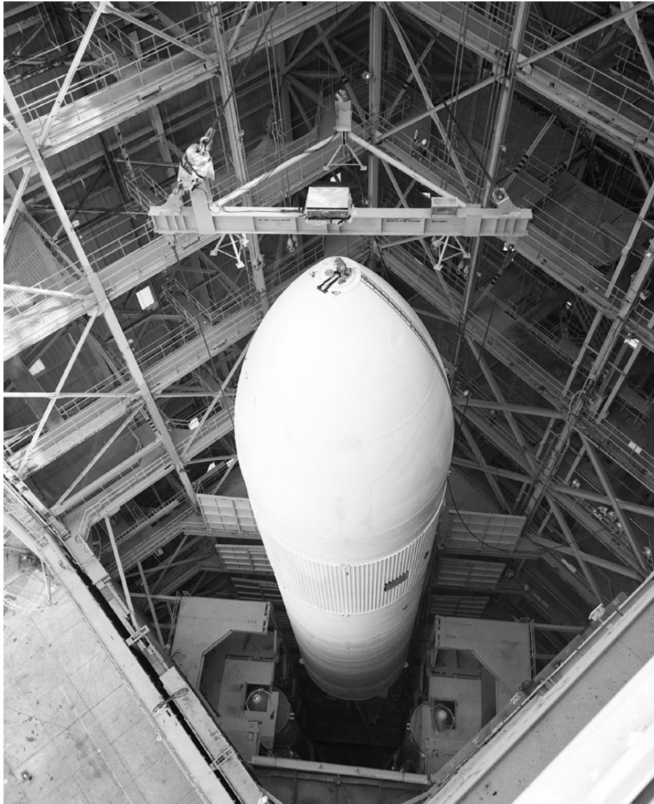
Figure D-4. Installation of ET into the Dynamic Test Stand (Building 4550) at MSFC for Mated Vertical Ground Vibration Test, September 29, 1978.
