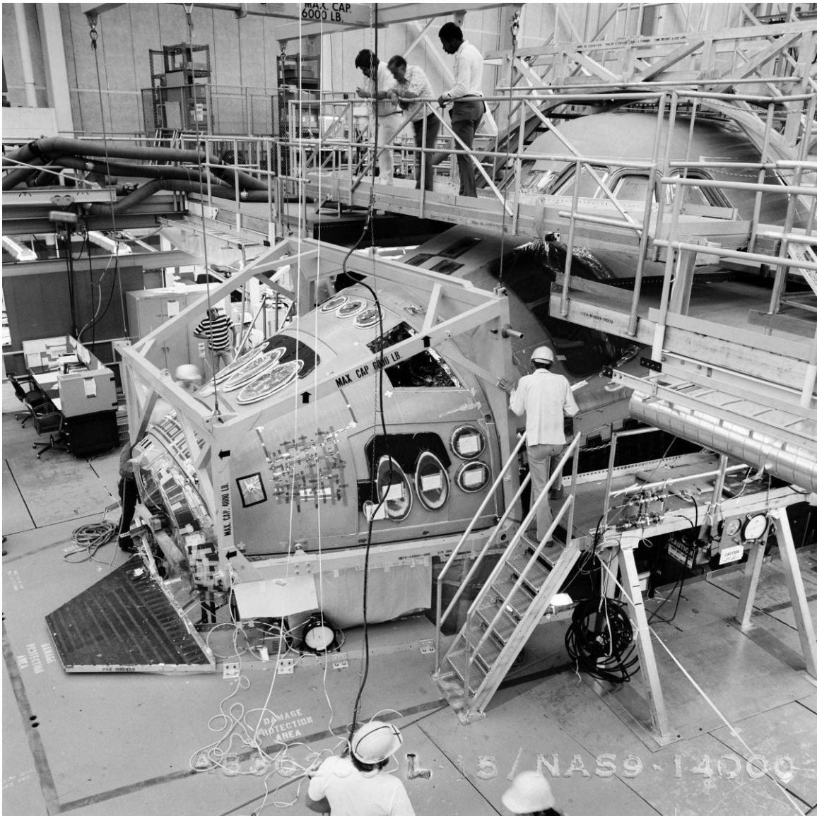
Figure B-41. Installation of Discovery's FRCS module in High Bay 2, AFP 42, February 9, 1983. Source: NASA, Johnson Space Center Image Repository, JSC2010-03410.
