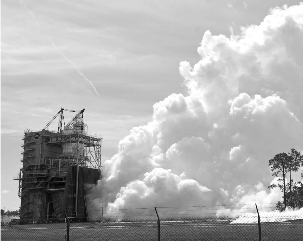
Figure C-12. A SSME undergoing testing on Stand A-2, camera facing southwest, March 30, 2009.
