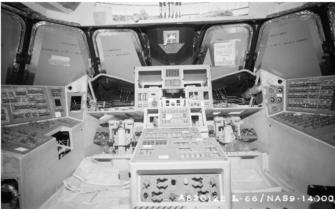
Figure B-40. Manufacturing progress on Discovery's flight deck in High Bay 2, AFP 42, January 25, 1983.
