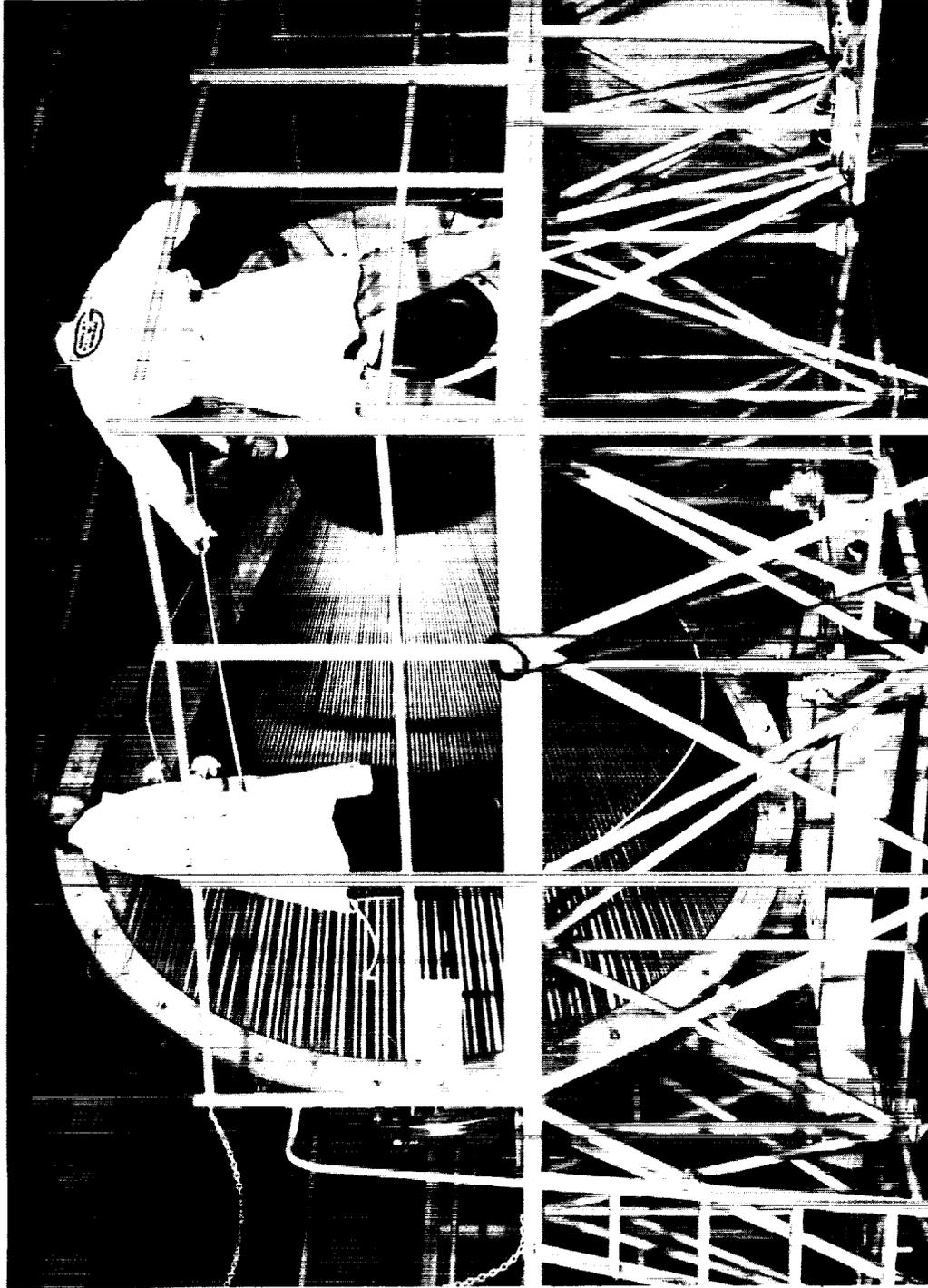
Figure 4. - M-1 Rocket Engine Project - Full-Scale (14 to 1) Combustion-Chamber Mandrel During Application of Tubing.
