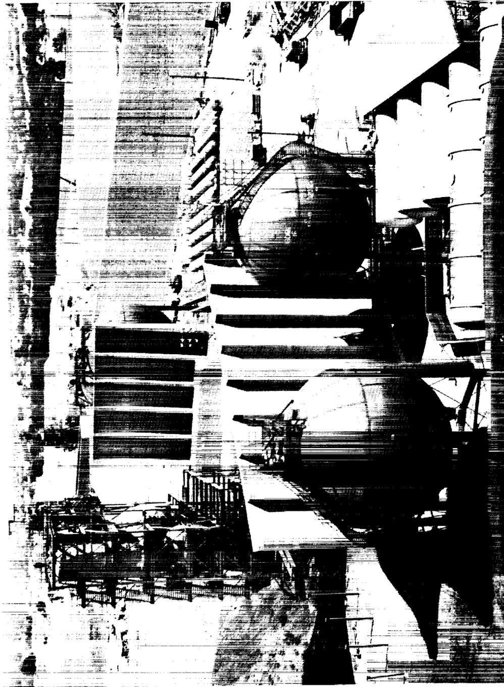
Figure 16. - M-1 Rocket Engine Project - Off-Stand Propellant Run-Tankage for Test Stands E-1 and E-3.
