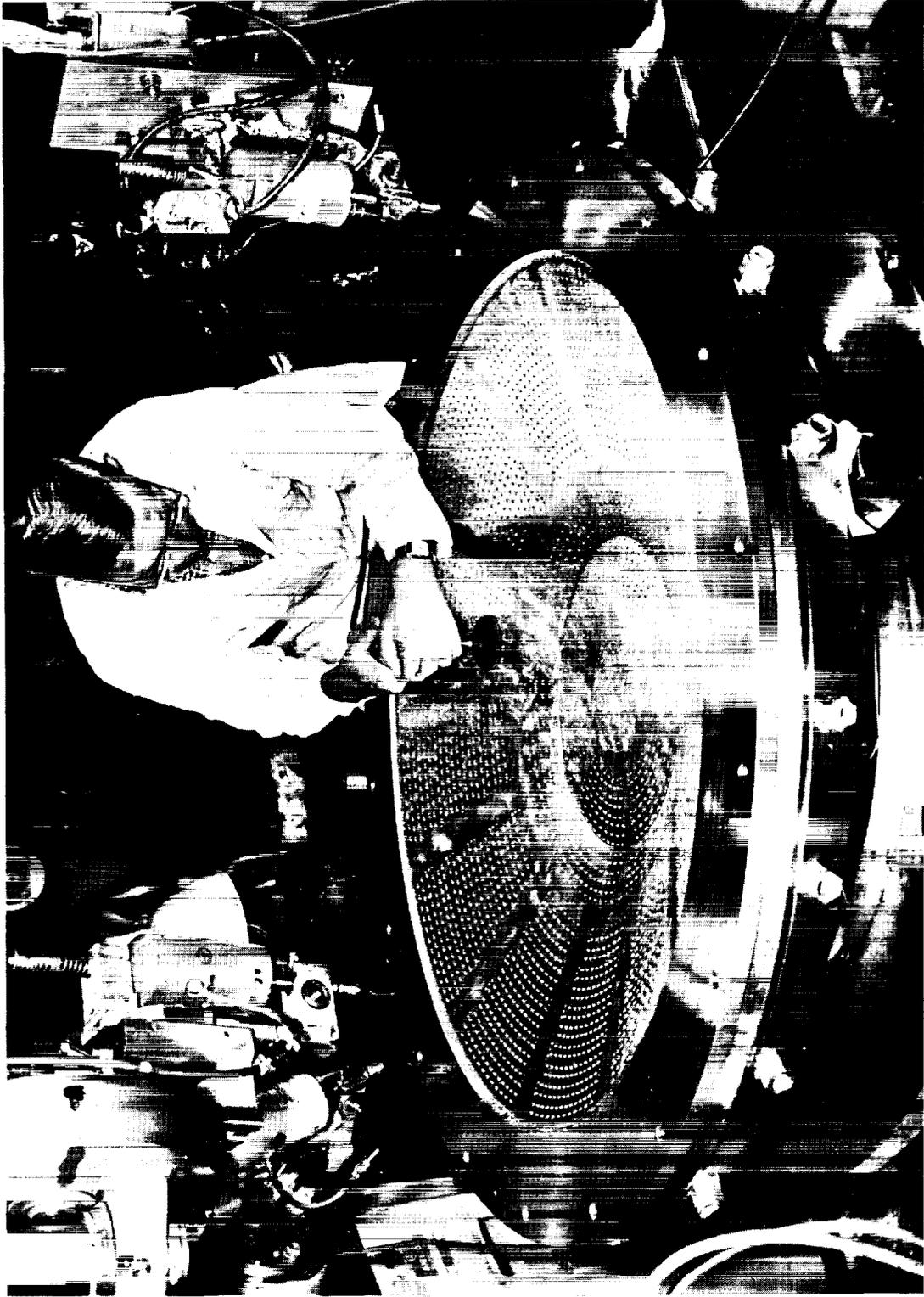
Figure 7. - M-1 Rocket Engine Project - Final Deburring of Thrust-Chamber Injector.
