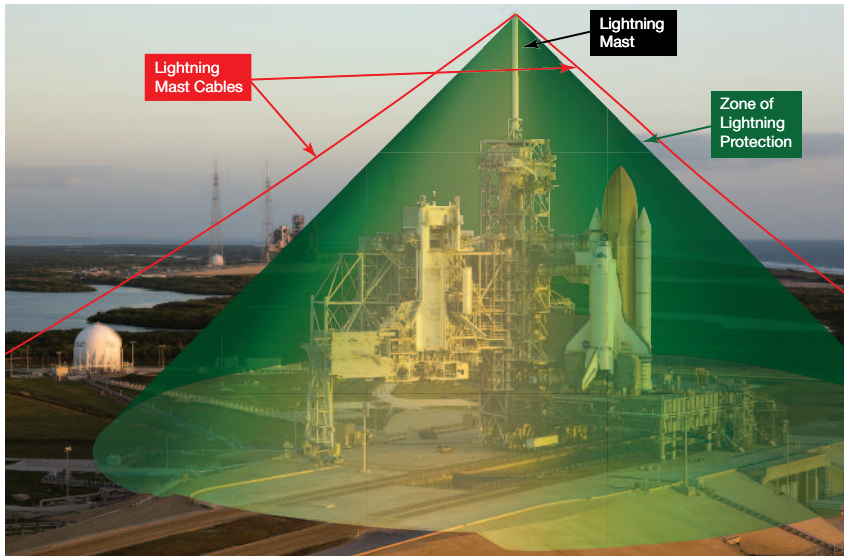
A grounded stainless-steel cable extends from the lightning mast to provide a zone of protection for the launch vehicle.
