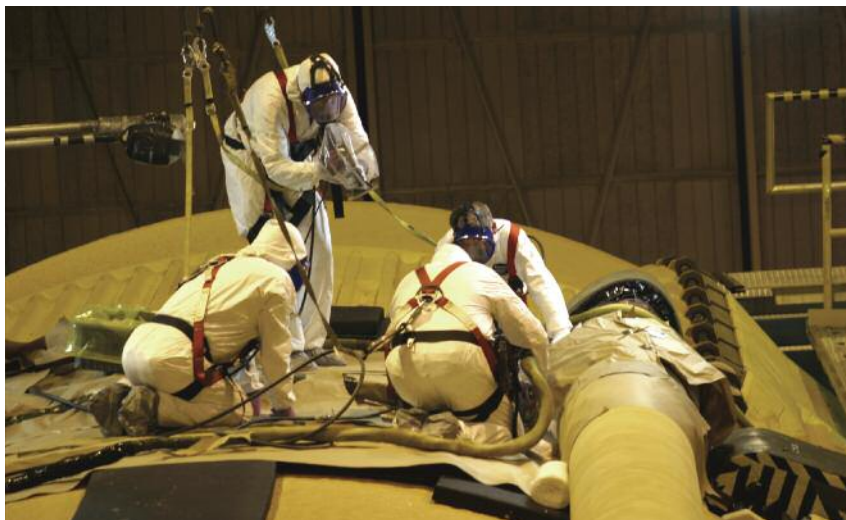
In what used to be a one-person operation, a team of technicians at NASA's Michoud Assembly Facility prepares to hand-spray BX-250 foam on the bipod attach fittings. The videographer (standing) records the process for later review and verification. A quality control specialist (left) witnesses the operation, while two spray technicians make preparations.
