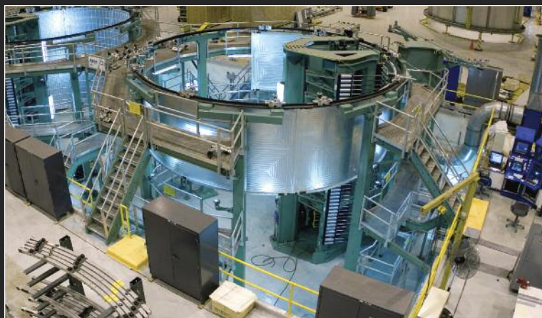
Friction stir welding units, featuring auto-adjustable pin tools, welded External Tank barrel sections at NASA's Michoud Assembly Facility in New Orleans, Louisiana. The units measured 8.4 m (27.5 ft) in diameter and approximately 7.6 m (25 ft) tall to accommodate the largest barrel sections.
