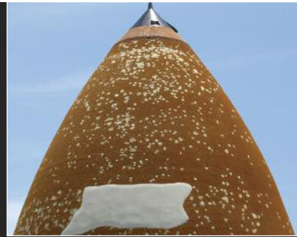
ET-124 damage repairs, post storm.
