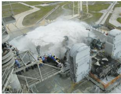
Water spray at the launch pad was used to suppress the acoustic vibration during launch.
