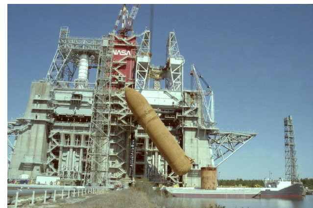
MPTA Tank Removal
